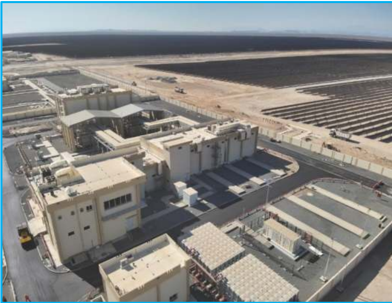
400KV MANAH IPP-1 GRID STATION
